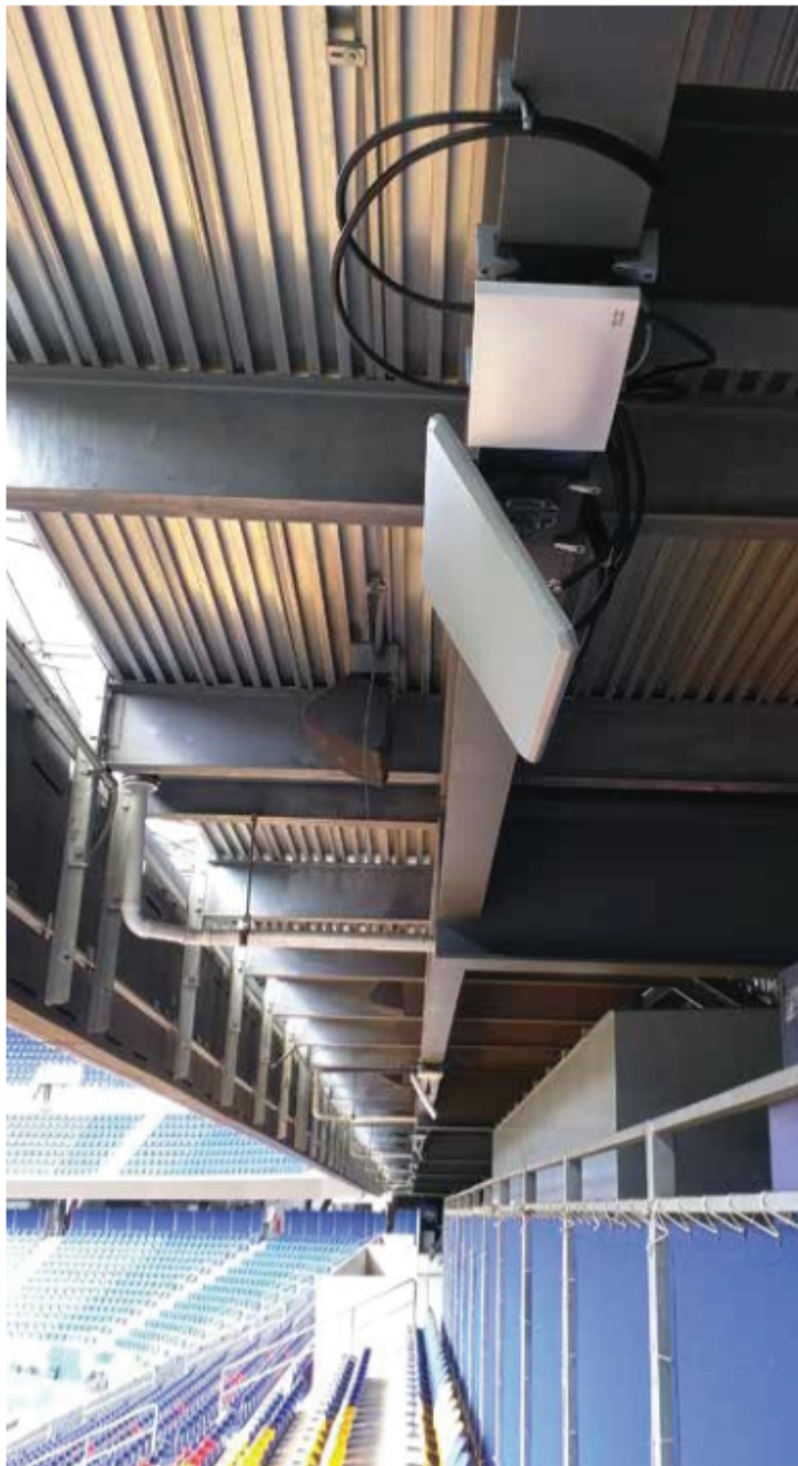
Safari Telecom created custom-built clamps and anchors for mounting the arena's APs.
