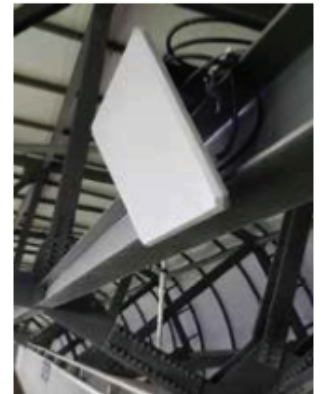
Red Bull Arena relies mostly on overhead APs to deliver Wi-Fi connectivity.
